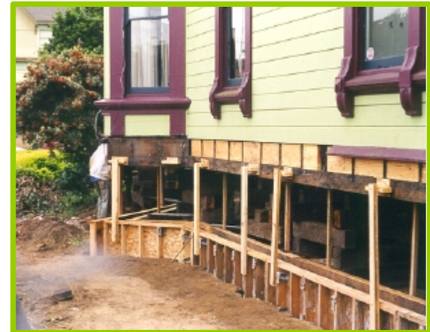
Seismic retro foundation
