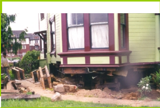
Seismic retro foundation
