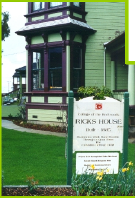
Seismic retrofit foundation and ADA access project
