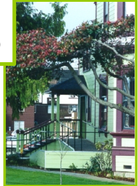
ADA wheelchair access ramp
