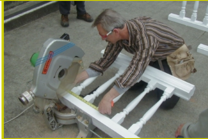
Trimming new balustrade to fit between reconstructed newel posts
