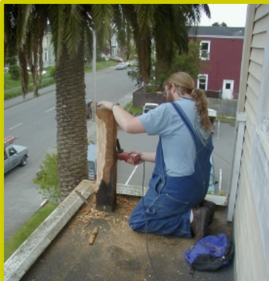
Repairing existing newel post for reconstruction
