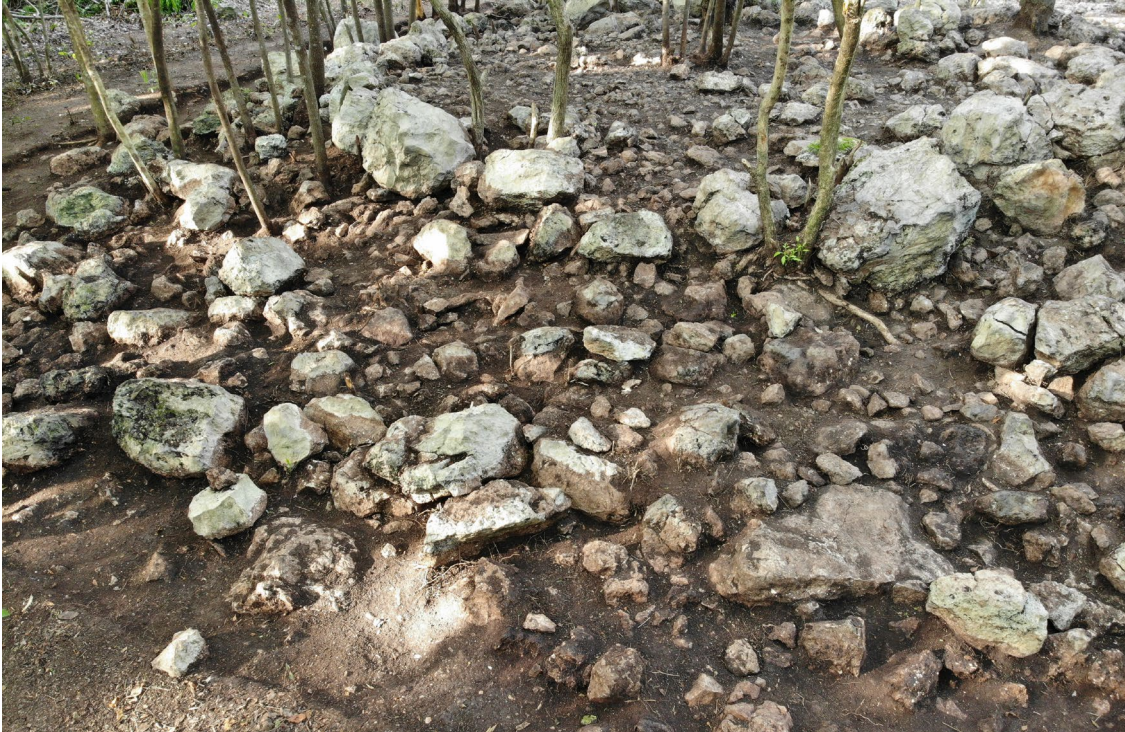
Figure 123. Sisal, Structure N1W3-1 (foundation brace) and Structure N1W3-3 (platform front wall)
